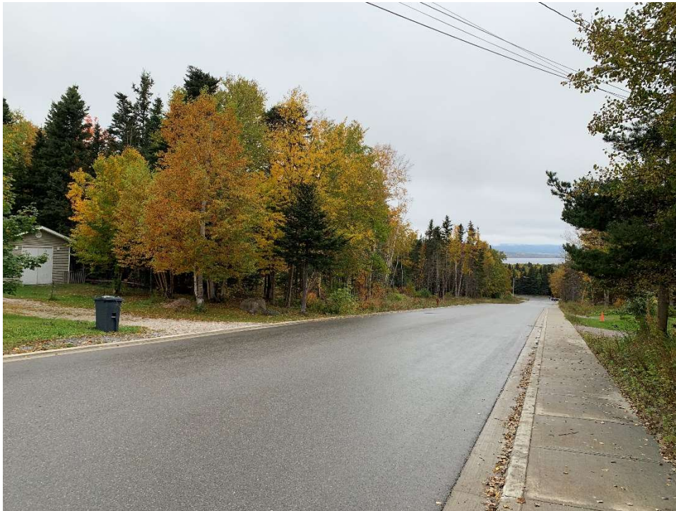
View looking northwest from Adam Crescent
