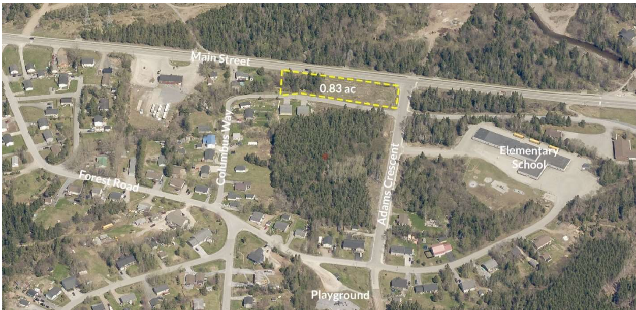
Image: Site Aerial View
