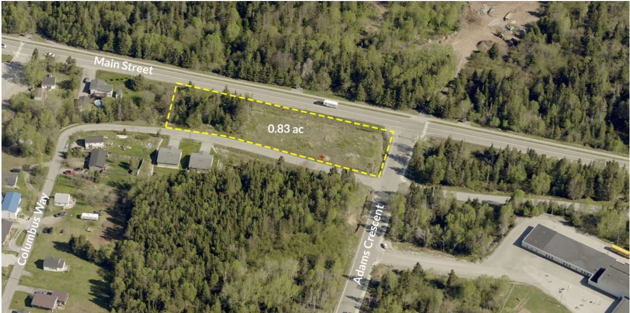
Image: Enlarged Site Aerial View
